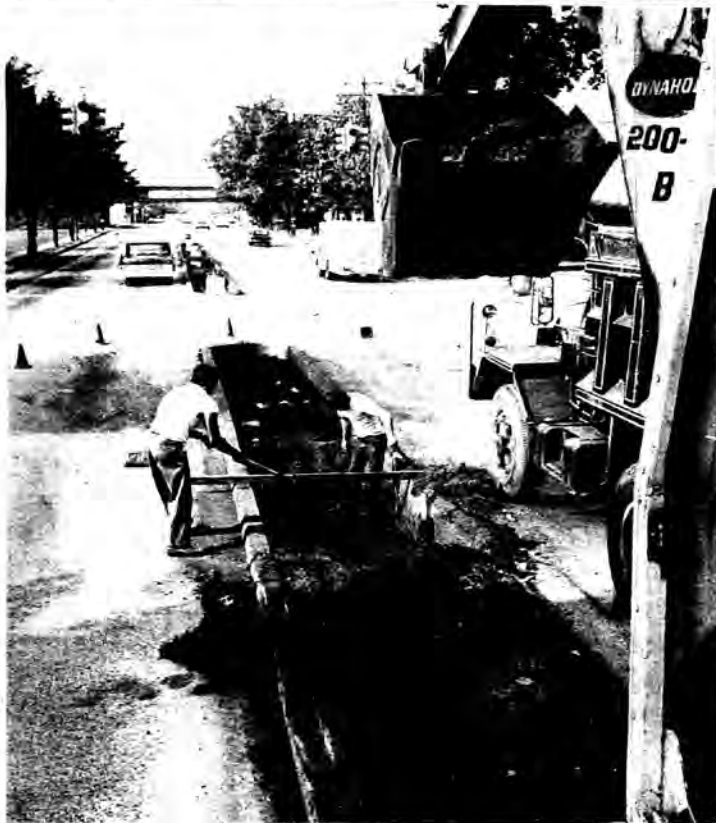
FOR A BETTER HICKSVILLE: Payer removing center mall from Old Country Road in Hicksville, the first step in a $335,880 Nassau County Department of Public Works project covering a 4,880-foot stretch from Railroad Avenue to South Oyster Bay Road. In addition to removing and paving the mall, the shoulders on each side of the road will be paved and left-turn lanes created by means of pavement markings. The changes will enable this section of Old Country Road, which has been the scene of 233 accidents in the past nine years, to conform in alignment, width and safety features to adjoining sections to the east and west.
