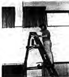
Walker Ritter washes down the walls of the Social Hall in preparation for a paint job.
