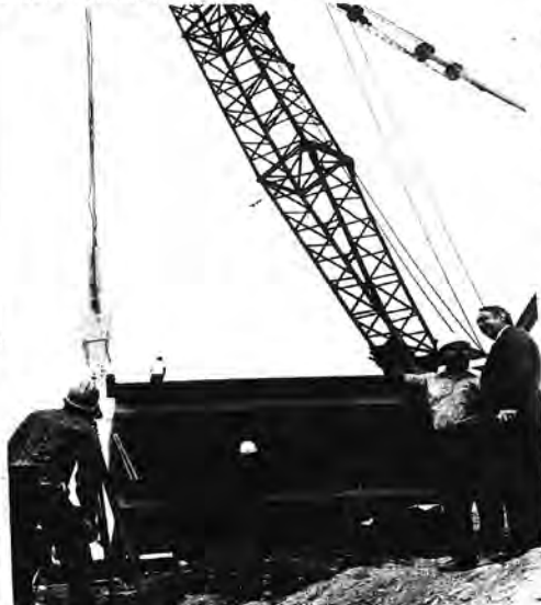
CONSTRUCTION PROGRESS: Oyster Bay Town Councilman Warren M. Doolittle, right, and Frank Capobianco job inspector for the consulting firm, Sidney B. Bowne & Sons, observe one of the pre-stressed concrete columns being lowered into place by crane at the new multi-level parking facility in Hicksville. When complete, the garage will provide parking for an additional 850 cars at the permanent location on Duffy Avenue and Newbridge Road. The project will be operated by the Department of Public Works public parking section of the Parks Division.
