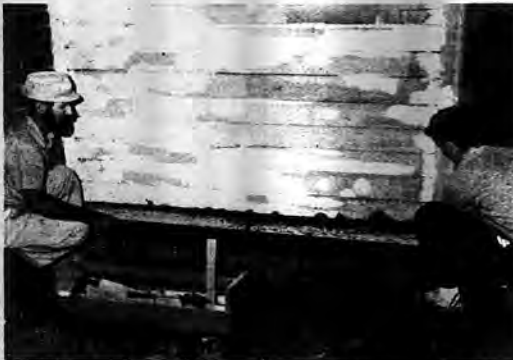
HELP WHEN NEEDED: Joe Bodner, Local Carpenters Union No. 1772, assisted by Kevin Sullivan replace damaged clapboards and molding at the Heitz Place Court House.
