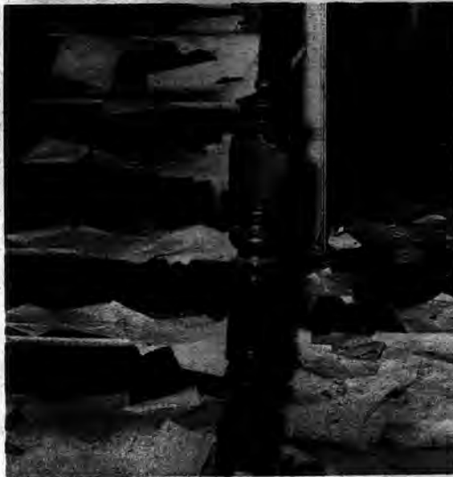
..WHEN WILL THOSE IN AUTHORITY TAKE CARE OF HICKSVILLE'S HISTORIC COURTHOUSE? Conditions at the Courthouse are rapidly going from bad to worse. It was reported to police this week that the front door has been broken open. Further vandalism continues.
