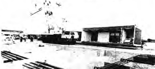
Modules leave the factory as self-contained units.
