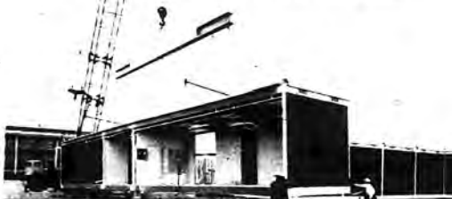
Modules can be joined to each other at any point on any wall.
