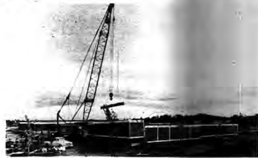
Final modules are placed in position.
