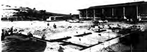
Permanent concrete foundations installed.
