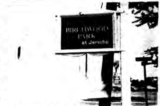
THIS ENTRANCE SIGN proclaiming "The Village of Birchwood Park at Jericho" was recently erected on the southeast corner of Jericho Turnpike and Merry Lane. Unable to secure local labor to do the installation work, the task was performed by the two highest ranking B.C.A. officials, Ed Petzholt and Sid Simon, President and First Vice-President, respectively. A similar sign was also placed on the southwest corner of Birchwood Park Drive and Robins Lane.
