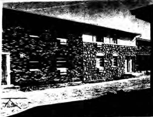
TENANTS MOVING IN... Attractive colonial styled facades highlight Bethpage Towne House, a new apartment complex erected by Jerry Spiegel Associates on Hicksville Road, between Central Avenue and Hempstead Turnpike, Bethpage. The 80-unit complex is now offering immediate occupancy.
