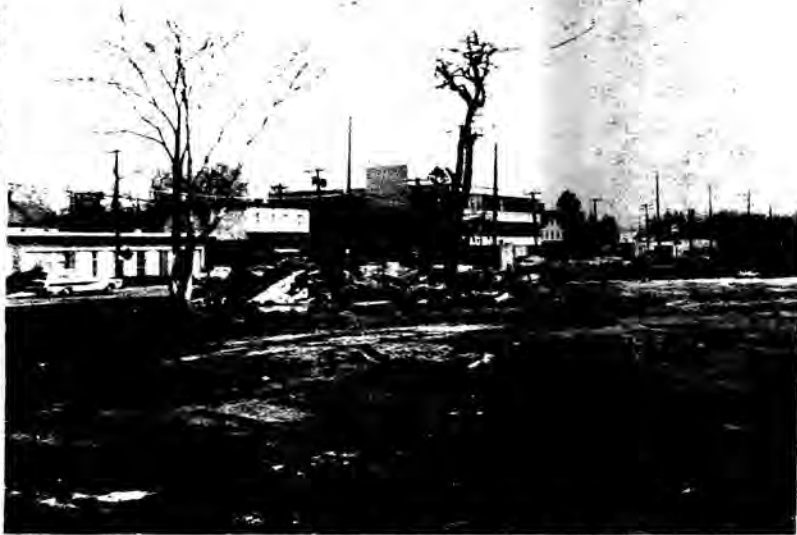
CLEARED LAND, the west side of Broadway from Cherry St. looking south to Old Country Rd., Hicksville, where acres of stores have been demolished. In the background are Seaman and Eisenmann, left, and Goldman Bros. (Herald Photo).
