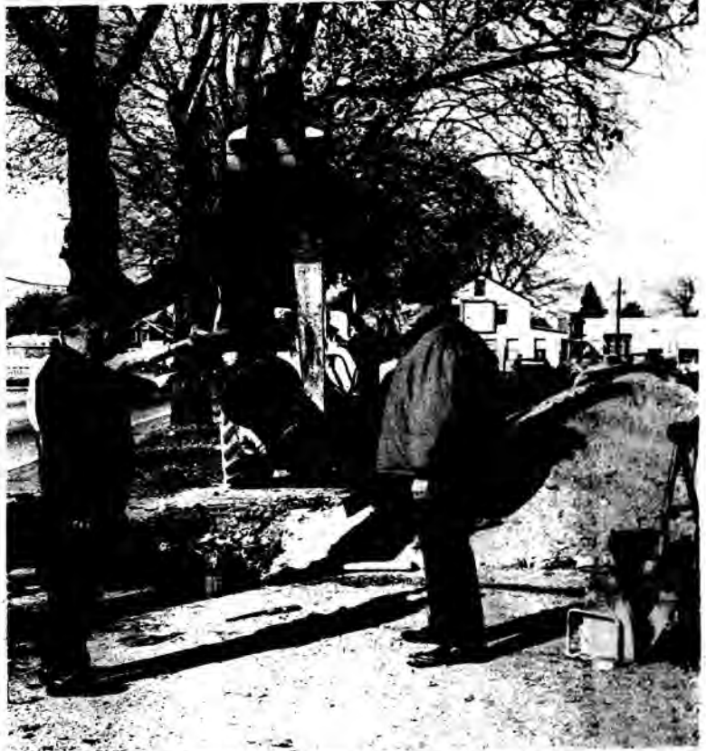
NEW GIANT TRANSMISSION MAINS are being installed on Broadway from Minnola Ave. north to Old Country Rd. by the Hicksville Water District to provide better pressure in the predominately industrial and business area of South Broadway before the widening of the state highway is completed, a saving for the future. Inspecting the progress of the work ordered by the Water Commissioners are Water District Superintendent Harold Hawhurst and Louis Dettloff of Karlison & Reed Constructors. (Photo by Frank Don Mallett).
