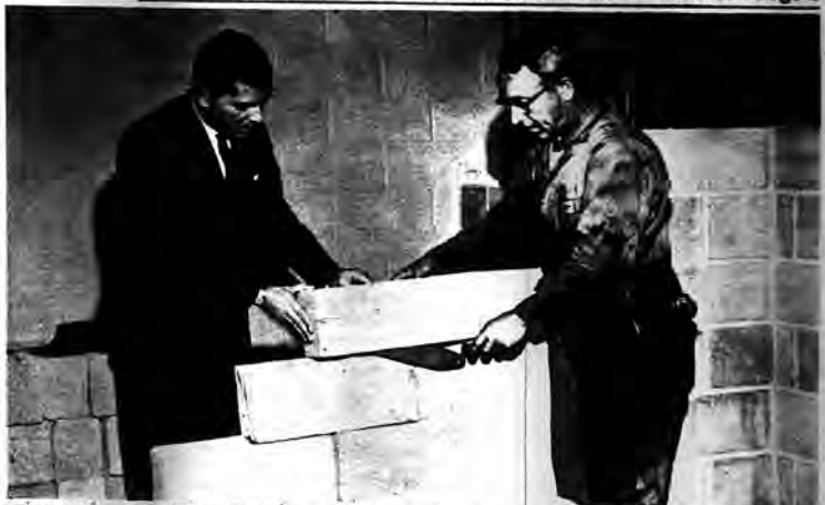
PUBLIC WORKS COMMISSIONER Herbert J. Simins of Jericho helps line up a cement block for a new wall as renovation of the interior of County Road Maintenance Garage on Cantiague Rd., Hicksville, gets underway. The $188,927 project will provide office space for the County Road Maintenance Division now located in the County Executive Building and one other Mineola-based County agency to be determined later. The moves will free space in Mineola needed for other County units.
