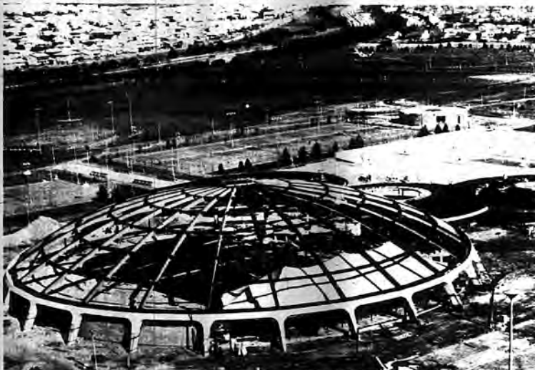
AERIAL VIEW, shows completed 360-ton steel frame for domed multi-purpose building prior to concrete pour for the roof. Several small circular flat-roofed buildings, interconnected with the major structure to provide shower and dressing rooms and indoor-outdoor dining facilities and a concrete deck swimming pool area, are seen in upper right background. The unique dome incorporates a design based on the principle of the Schwedler dome, developed during the nineteenth century, whereby the entire dome is structurally independent of the precast concrete compression ring beneath it. The entire dome, weighting 3600 tons including steel work and concrete, is supported by 24 vertical steel ribs, each anchor bolted below to one of the tapered precast architectural concrete tees, or columns. The structure, 56 feet high and 210 feet in diameter, is reportedly the largest of its type in the nation.
