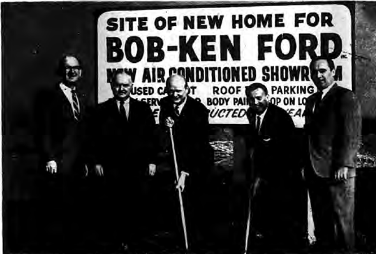
GROUND BREAKING of new Bob-Ken Ford, Inc., Bethpage Rd., Hicksville, took place recently. Building will have air-conditioned showroom, roof top parking, and complete facilities for parts, service, repairs and paint shop. From left are Brian Medler, sales manager, N.Y. District Sales Office Ford Division; Conrad Favelle, contractor; Bob Wallace, Ken Gilkes, John Mallen, New York manager dealer development, Ford Motor Company. Wallace and Gilkes, partners in Bob-Ken Ford represent over 65 years of quality car merchandising.
