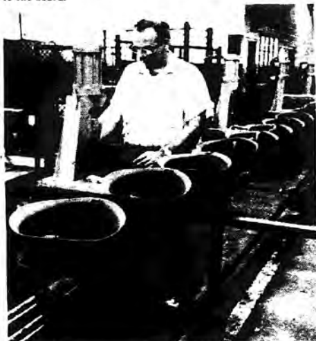
STEEL CHAPEAUS —The first helmets to be ordered by the government since 1958 move along the production line. The style of the "steel pots" is virtually unchanged from World War II models. Borg-Warner Corporation's Ingersoll Products plant in Chicago will make 732,000 of the helmets under contracts totaling $2.6 million.
