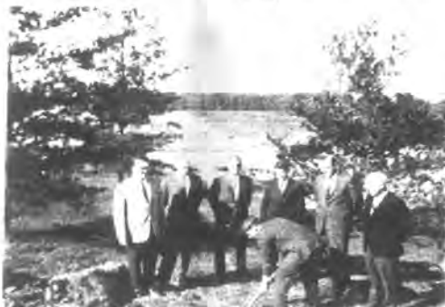
MARC MILLER, President of the Jericho High School Student Council takes the first shovel full of soil at the site of the new addition to the High School. Looking on approvingly are the members of the School Board and Dr. Heller, principal of the High School.
