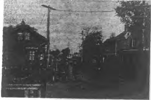
WAITING ROOM of Hicksville RR station as it looked about 60 years ago when it stood on the north side of the tracks between Broadway and Jerusalem Ave. In those days there were gas lamps, flower gardens, glazer bread on the roof and iron-wheeled luggage wagons. The back of Herzog's store on Herzog Pl is visible in the right of center background.
