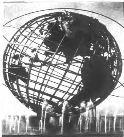
UNISPHERE, symbol of the N.Y. Fair theme, "Peace Through Understanding," was engineered and built by United States Steel. The world's largest model of the globe, the stainless steel UNISPHERE rises 12 stories and weighs over 900,000 pounds.
