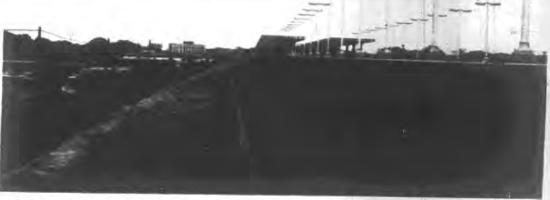
JUST WAITING for the trains and commuters is the new high level Hicksville Rail Road station. Top picture shows the middle track as it looks from the extreme west end of the long, long platform. At the bottom, from the same position, are the new rails with the present temporary tracks and station at the extreme left. The Professional Building is in the background. (Exclusive Herald Photos by Frank Don Mallett.)
