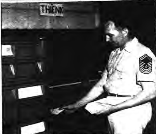
MASTER SERGEANT Vincent Van Houten of 21 Lawrence St., Hicksville, runs punch cards thru the IBM sorter which sorts data cards at the rate of 800 a minute. Van Houten is a data processing specialist in the Comptroller's Section of the 106th Aeromedical Transport Group, New York Air National Guard, at Floyd Bennett Field, Brooklyn. Master Sergeant George Stenzler of 8 Prospect Pl., Plainview, is also a key man in the comptroller section.
