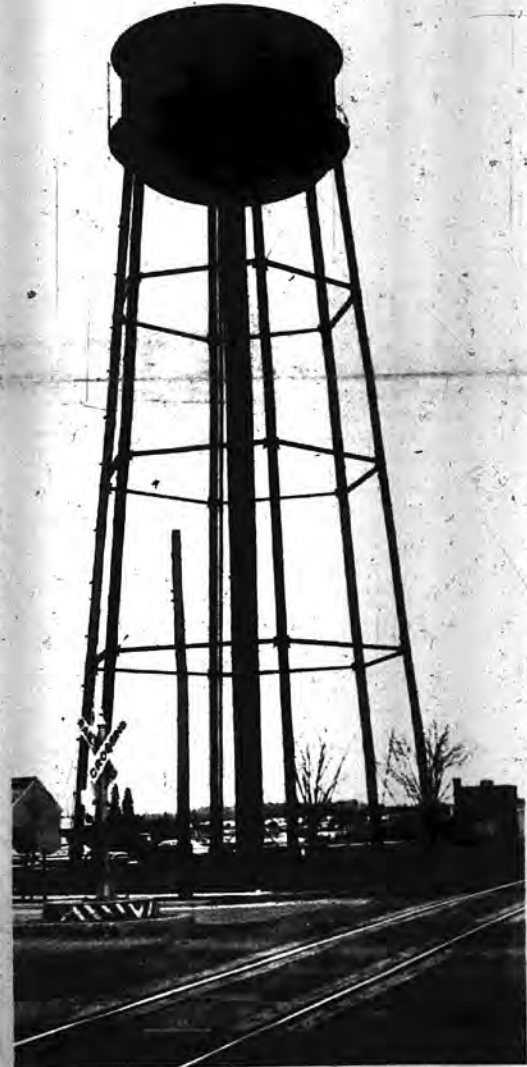
VICTIM of the Hicksville RR grade crossing elimination program will be the "tea cup", first elevated storage tank of Hicksville Water District. Before the week is out the 146-ft. tank will be gone.
