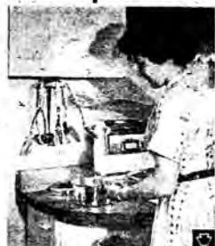
"LET THERE BE..."—A three-cathode xenon light source, believed to be the first multiple cathode unit built, is being tested by U. S. Army Engineers as a means of lighting a greater area than now possible. In a searchlight, the three-in-line arcs (insert, upper right) gives the unit high candlepower and a horizontally spread beam without spread losses.
