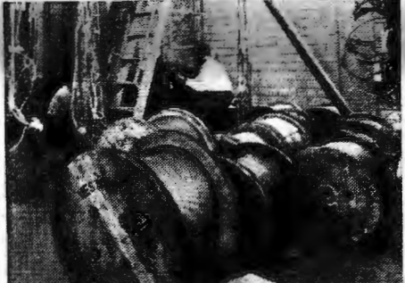
MILLIONS of electrical connections have had to be made to interconnect the telephones served by LEvittown 3 and 9 and tie them into the vast telephone system.
