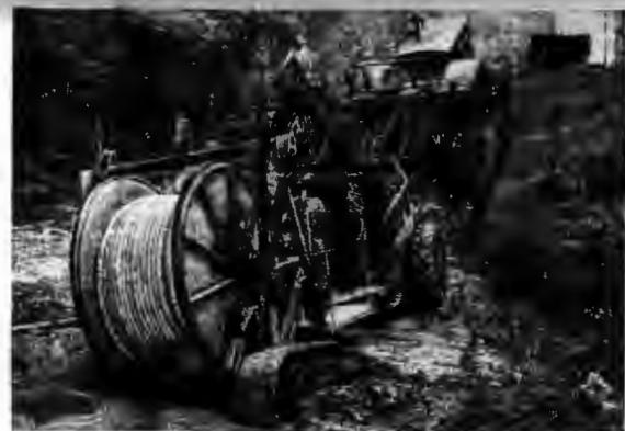
**1,800 VOICES IN THE EARTH.** A coaxial cable, capable of carrying 1,800 Long Distance telephone conversations at the same time, is shown here being laid underground by tractor train. Coaxial cables are a vital part of the Long Distance network, which is so busy these days with defense calls.
