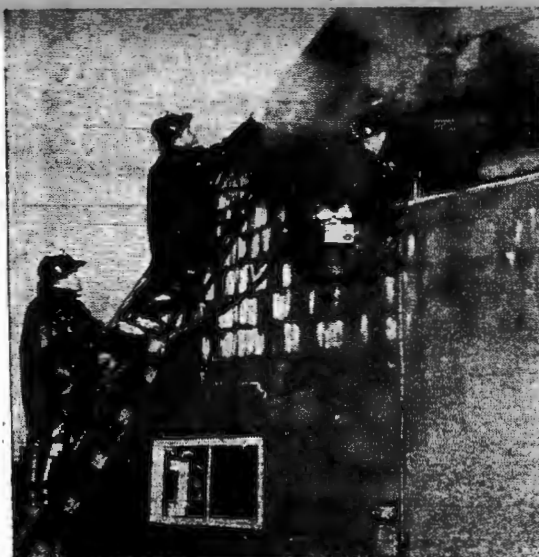
UP A LADDER are Constantine Cotsonas and Dick Meditz of the Hook & Ladder Co. with George Frey of Chemical Co. 3 inside the attic at the Schwartz home, 17 Walnut Lane, Hicksville, where considerable damage was caused to the second floor on Sept. 8. More than 50 men of Hicksville Fire Dept. under Asst. Chief Larry Hottle fought the fire for two hours. (Herald photo by Frank Mallett).
