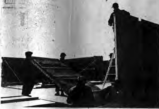
WINDOW PANEL being set in place at Hicksville's temporary school building site
