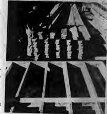
PRECUT and formed rafters and interior wall panels on location
