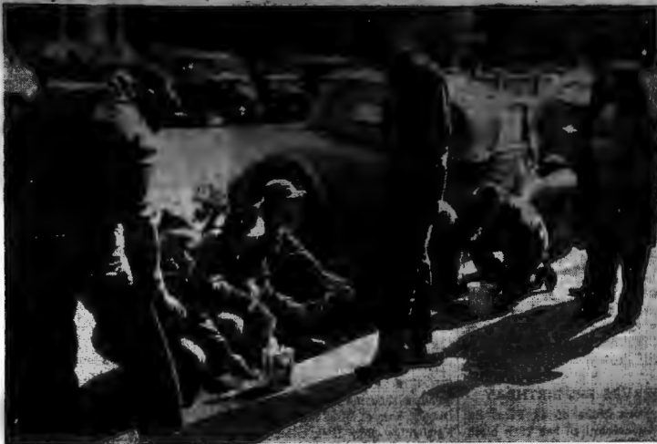
LOADING ONLY —Members of Hicksville Lions Club, with the official permission of the State Public Works Dept., spent a Sunday morning marking four loading zones on Broadway which have proven to be "fine traps" for unsuspecting motorists. Here they tackle the curb painting job in front of Firestone, 114 Broadway. Standing, left to right, are William Stakley, who watches for a spot of paint on his
