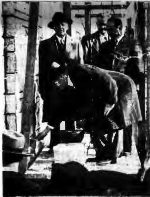
G.F. WENNAGEL handles the trowel at the ceremony of laying the cornerstone for the new Methodist Church. Rev. Cranston Clayton, pastor, looks on (centre, standing) with two stone mason contractors. (Mallott Photo)
