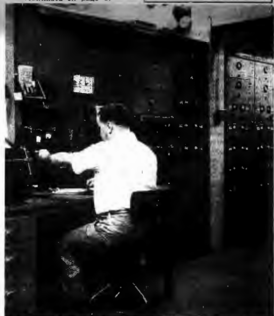
CONTROL BOARD of the Press Wireless Inc. transmitter station on Cantiague Rd. In 1945, when this picture was taken, the Hicksville radio station was handling more than 100,000,000 words of radio telegraph traffic in a year, using about 30 transmitters.
